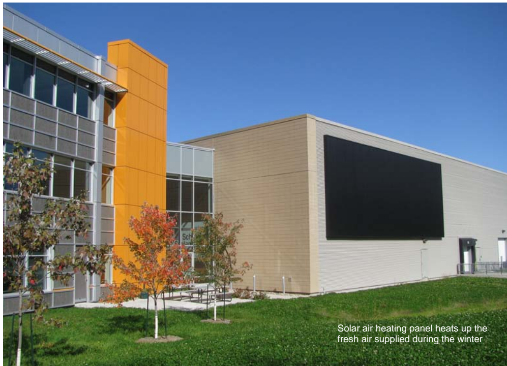
Schlüter® Systems Canada - 6100 m 2 building located in Ste-Anne-de-Bellevue, QC- LEED® Gold certification
