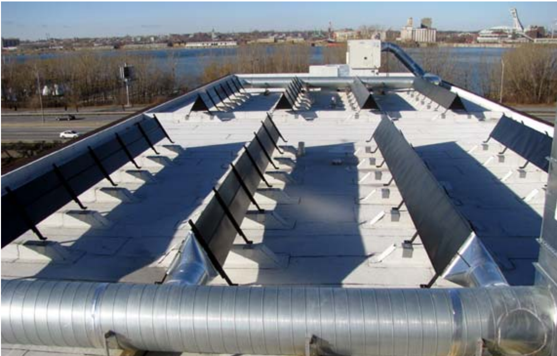
80-unit "Bord de l'eau" project in Old Longueuil, Quebec - LEED® Canada for Home Certification
